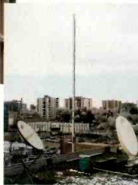
From downtown Denver, KMGH-TV broadcasts a low-power DTV signal using a Scala antenna mounted on its roof, and Larcant transmitter installed in the penthouse of its five-story building.
